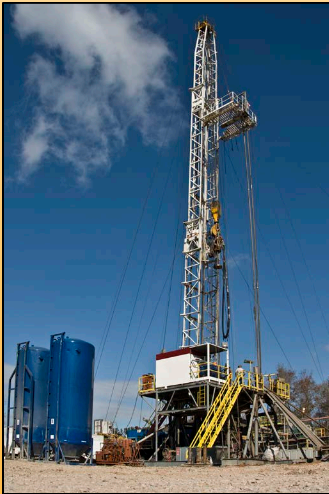
Drilling operations in the Eagle Ford Shale
