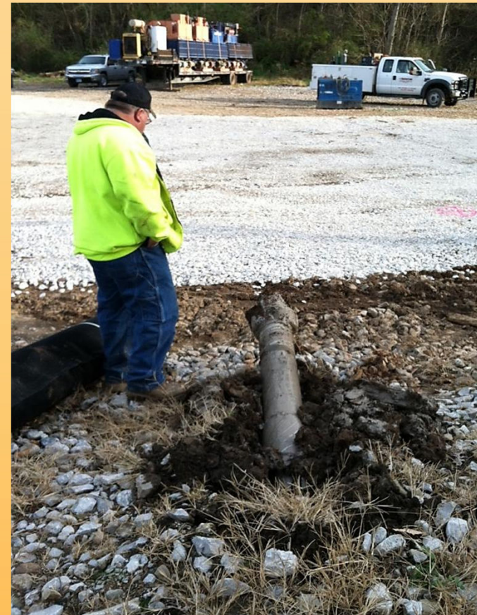
Ohio River Bore into Ohio
