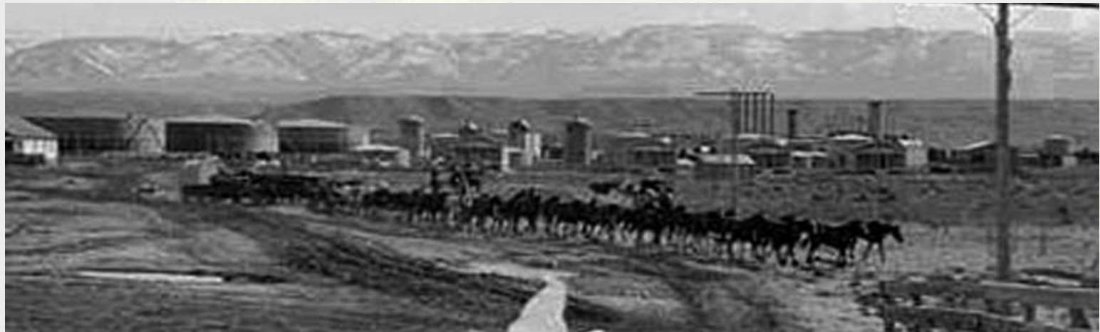
Transporting equipment to Salt Creek.
