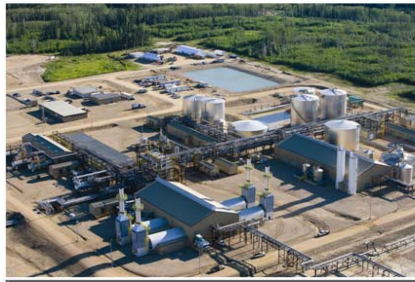
Surmont 1 Central Processing Facility
