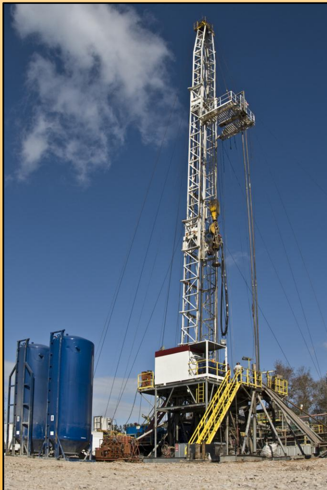
Drilling operations in the Eagle Ford Shale
