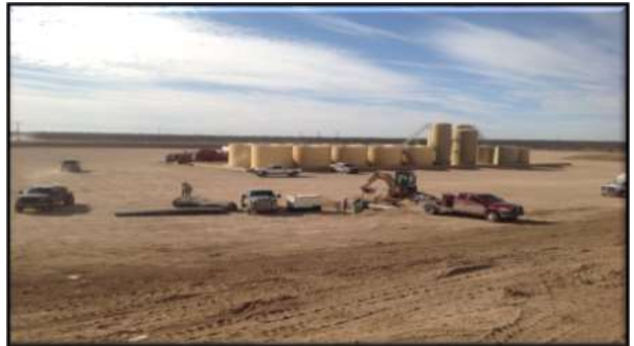
Water Recycle Facility (Under Construction)
