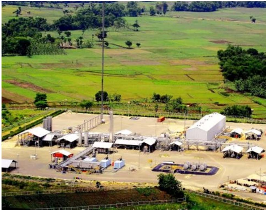
Banyu Urip Early Production System Gas and Oil Separation Plant
