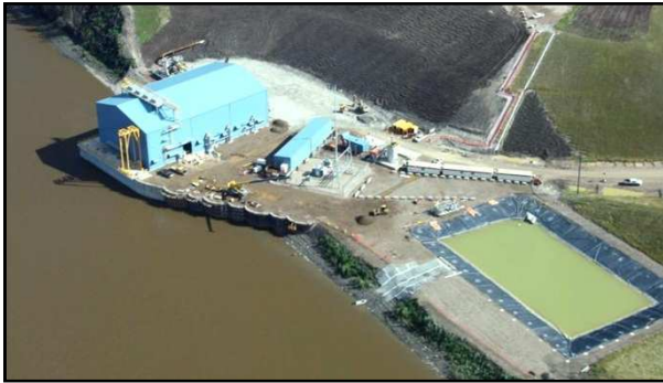
River water intake
