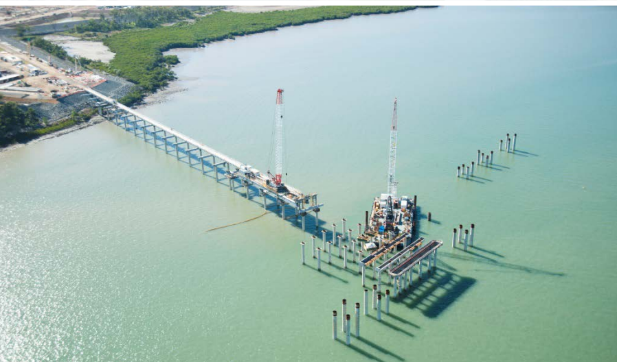
All of the LNG jetty bents have been completed
