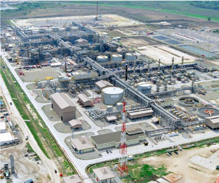
Banyu Urip Central Processing Facility, Indonesia
