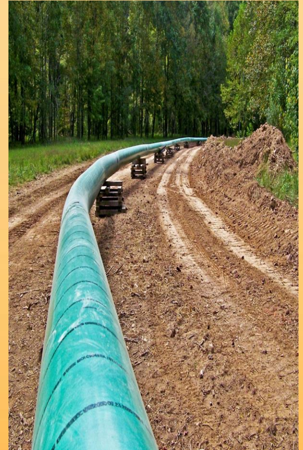
Strung Pipe Before Being Lowered
