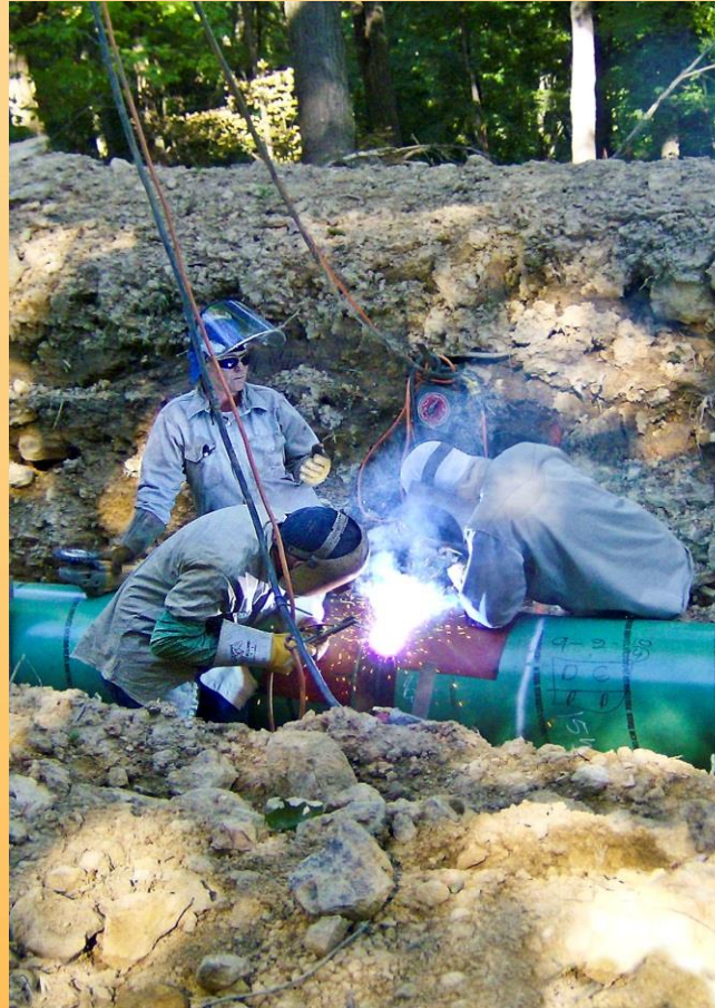
Welding Up Pipeline Connection
