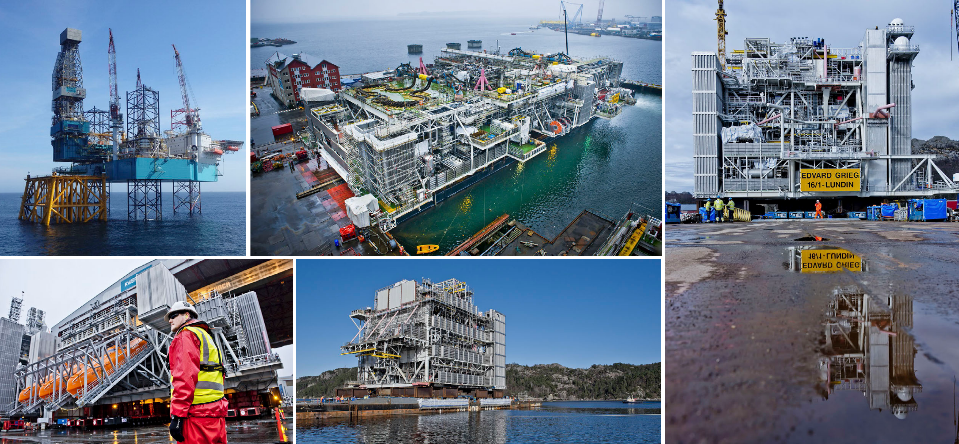
Edvard Grieg development drilling and topsides load-out
