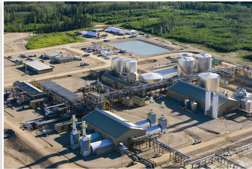
Surmont 1 Central Processing Facility
