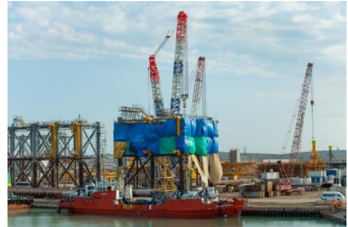
Construction of an offshore platform.
