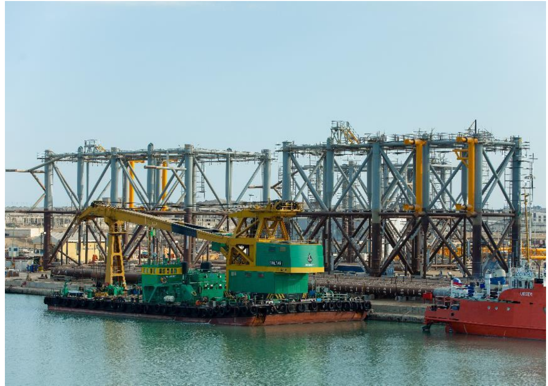
Fabrication of an offshore platform.
