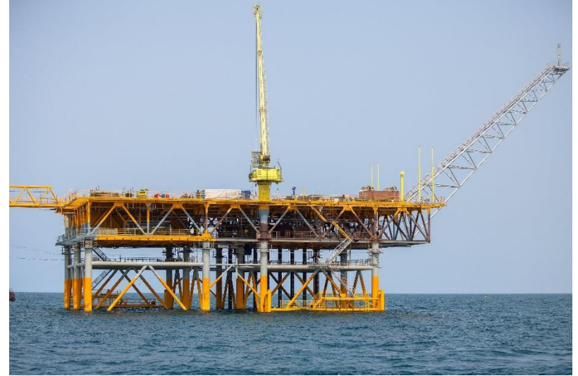
The Dzhygalybeg (Zhdanov) offshore platform.
