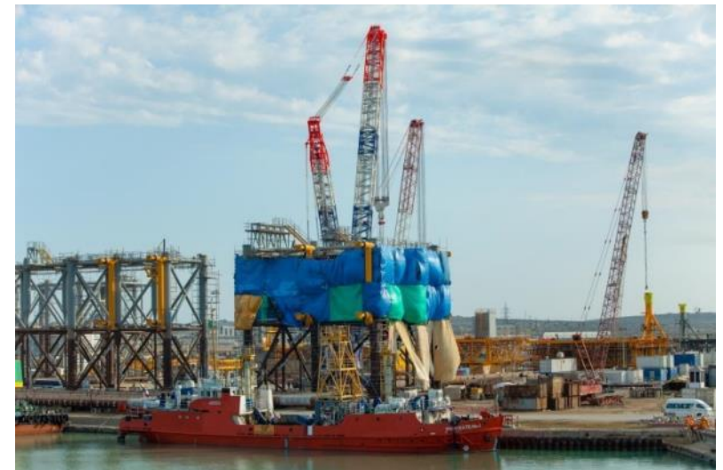
Construction of offshore platforms at the harbour area.
