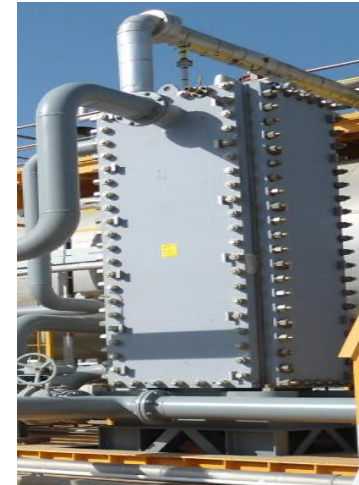
Preheat exchanger and degasing boot.
