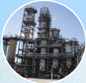
First lube oil hydrofining
