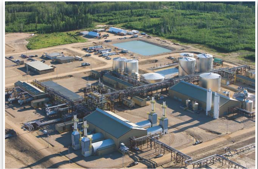
Surmont 1 Central Processing Facility
